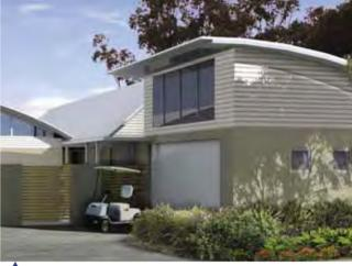
Horizontal timber slats offer a good alternative to solar protection and eave overhang.
